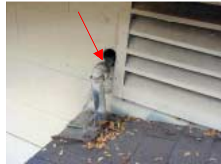
seal hole at right side exterior wall
