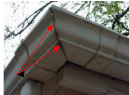
damaged gutter
