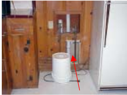
wall opened below washer plumbing
