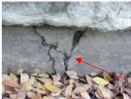
slab crack
