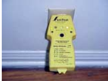
grounded outlet in living room
