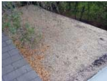
carport roof covering
