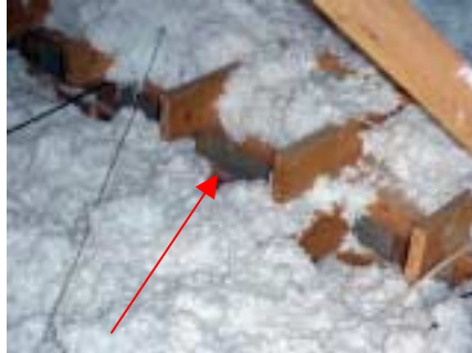
missing fire stopping and insulation
