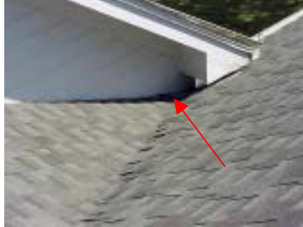
potential leak area
