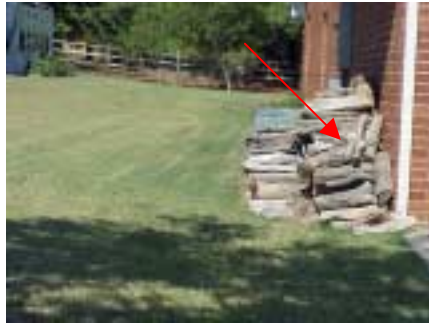
remove wood (conductive to termites)
