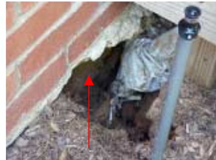
void in soils near rear porch
