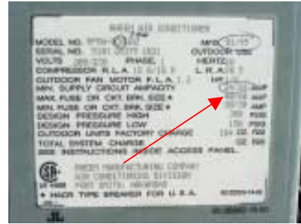
condensing unit data plate
