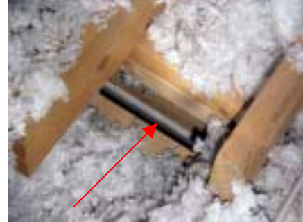
missing fire stopping and insulation
