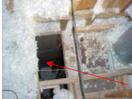
missing fire stopping and insulation
