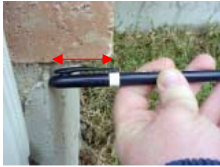
excessive overhang at right side
