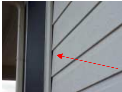
seal gaps at exterior
