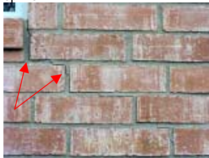
separation at left exterior (monitor)
