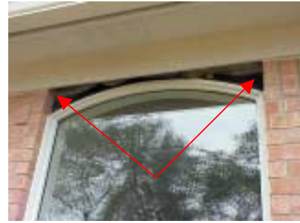
brick veneer missing above window
