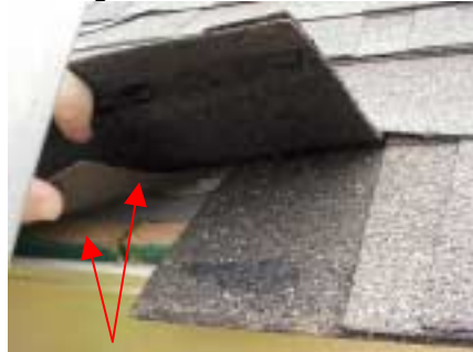
starter course wrong and felt cut short
