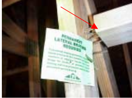
brace not properly installed
