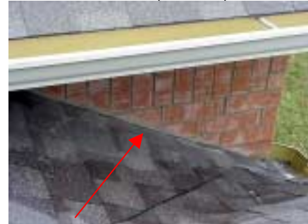
non-conventional method of flashing
