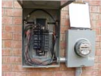
electrical panel at left exterior
