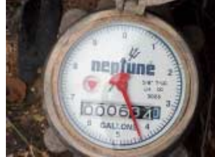
no signs of hidden leaks at water meter
