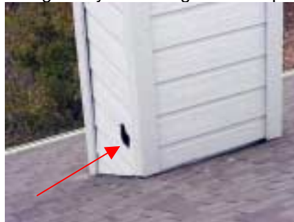
combustion air cap missing at chimney
