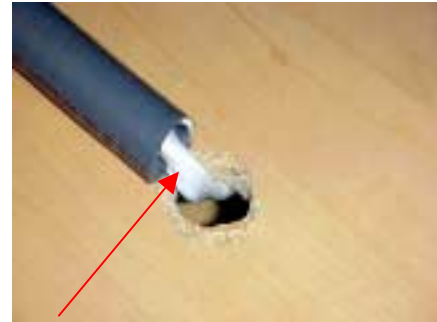
conduit not properly installed
