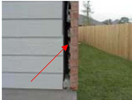
rear left corner not finished out
