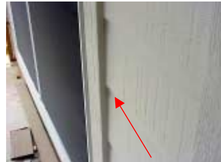
example of properly sealed gaps
