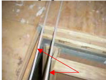
wires not properly secured
