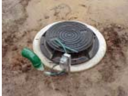
rain water collection system?
