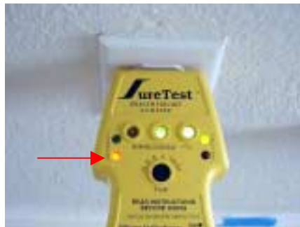
excessive voltage drop
