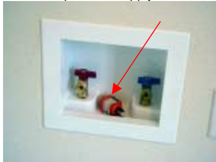
remove drain cap at washer
