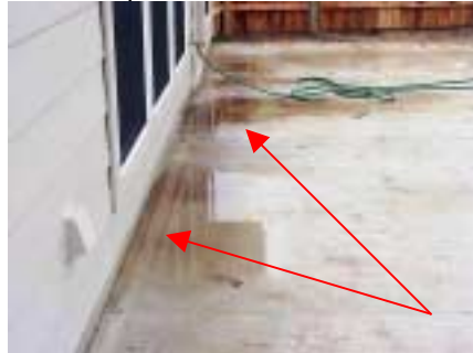
improper drainage at rear patio
