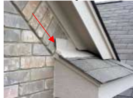
missing counter flashing above front entry
