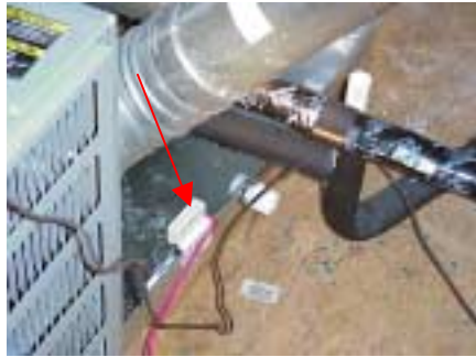
extend drain from pan to exterior
