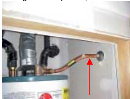
T&P drain line does not gravity drain
